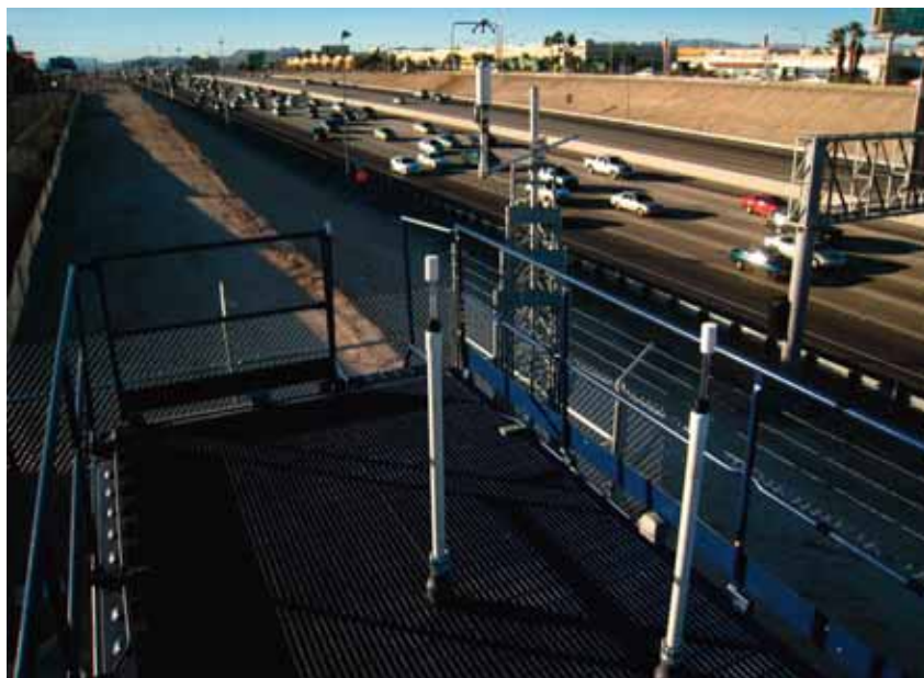
Figure 1. Near-road air monitoring station—dual sampling manifold system; quartz manifold for VOC sampling and pyrex manifold for gaseous criteria pollutants sampling.
